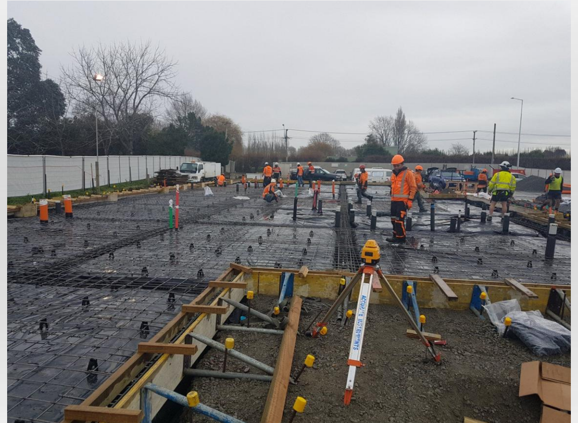
Mr Box Installation, Christchurch
